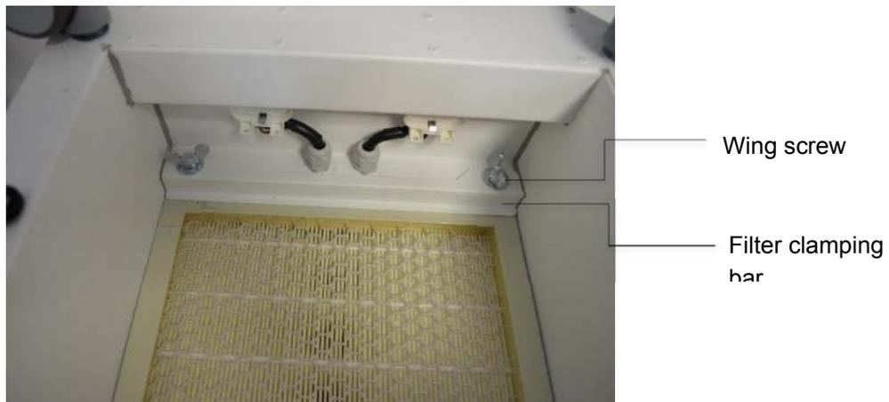
Abb. 28 Wing screws and filter clamping bars
